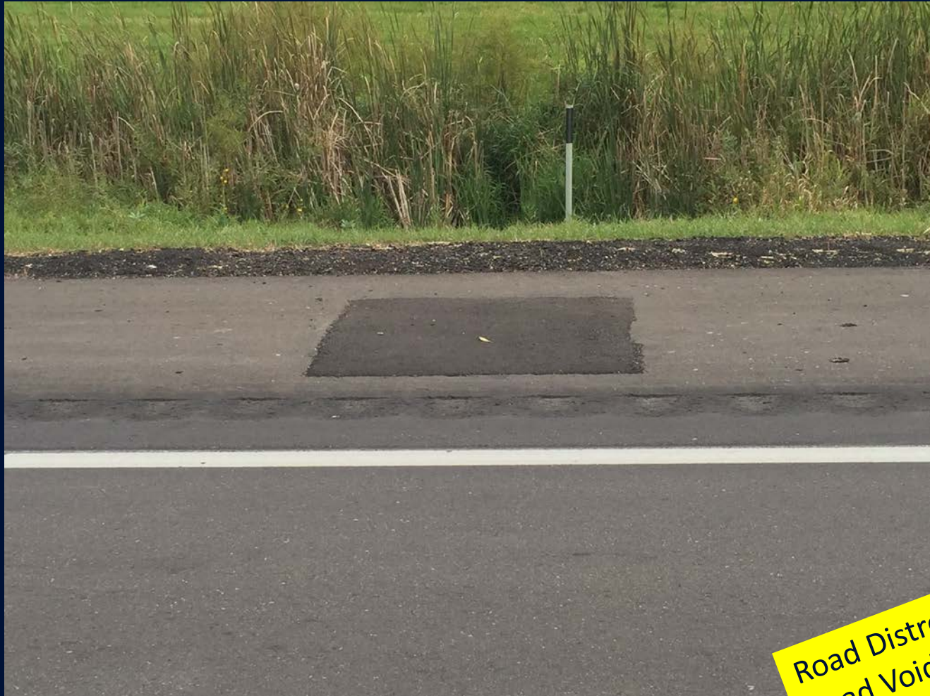
Photo by HydInfra Inspector Brad Fredin October 2018, MN55 project
