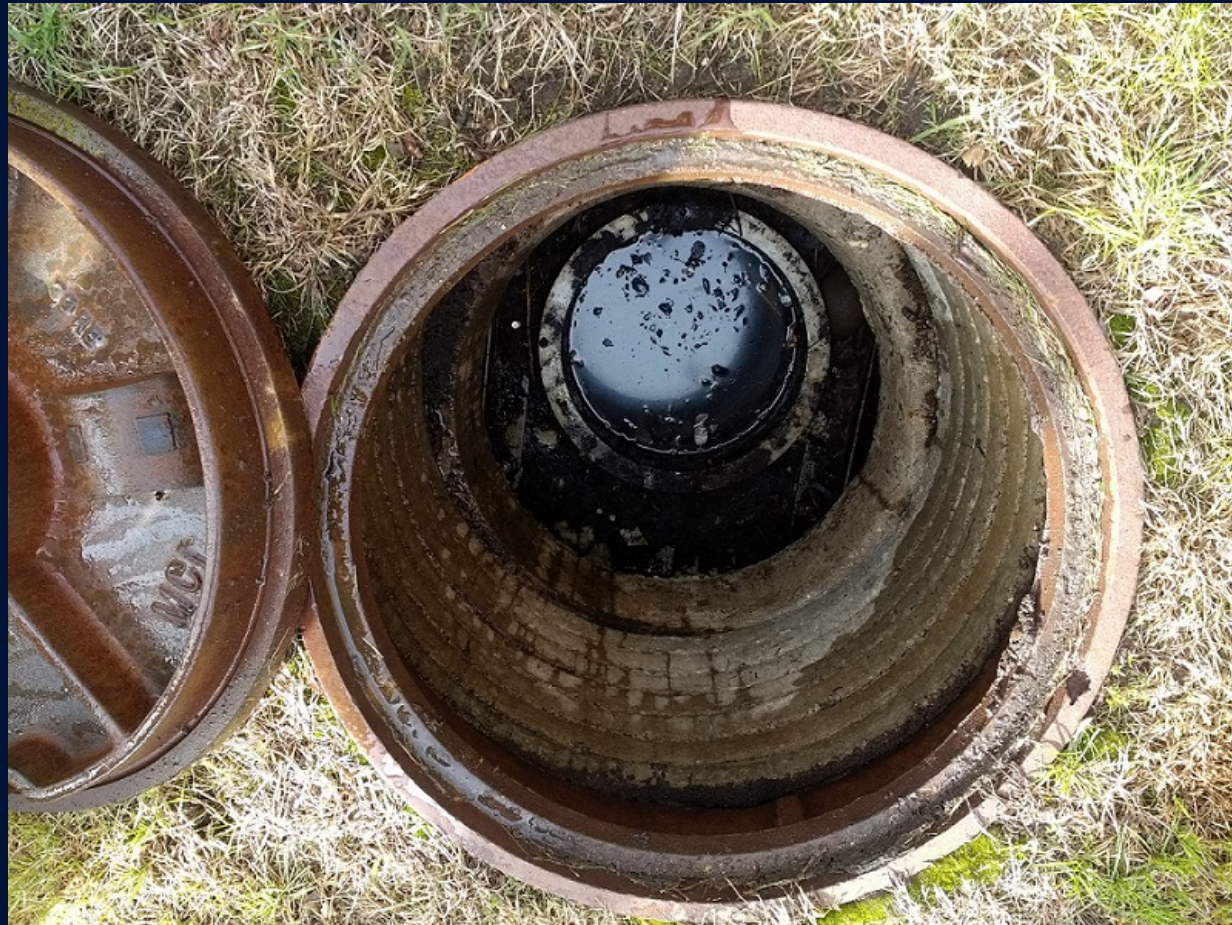
Structural Pollution Control Device, Separator on MN 23 D8
