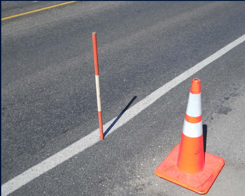
D6 Jacked Pipe creates road void 27SEP2011 – Rob Coughlin
