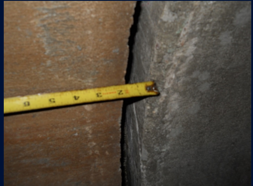
D6 Jacked Pipe creates road void 27SEP2011 – Rob Coughlin
