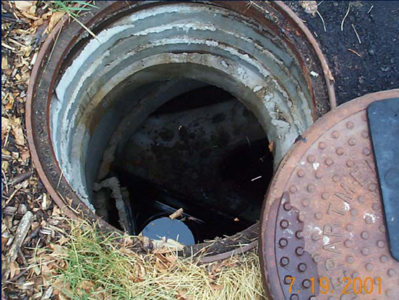
Manhole (solid cover) with 3 rings
